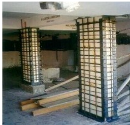
Fig. 1: Construction Techniques for Column Jacketing.
