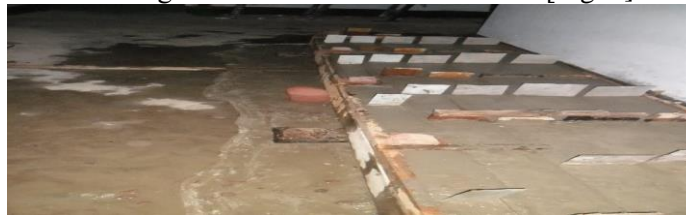
Fig. 1: Casting of pre-cracked beams inserting steel plates
