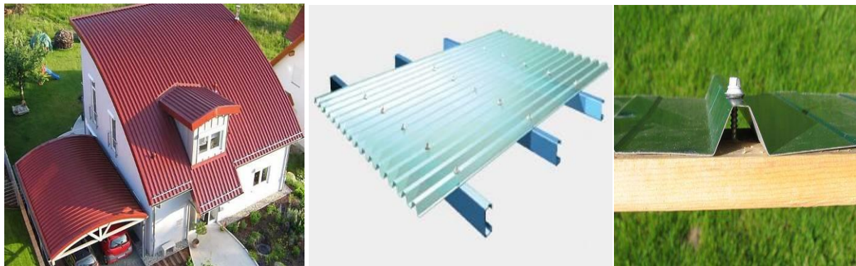
Fig. 1: Field application of profiled steel sheet using bolted and screwed connections
