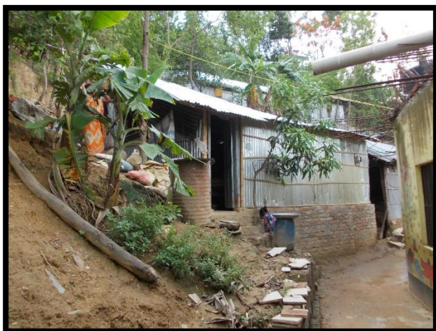
Fig.3: Vulnerable house besides hills Source: Field Survey, 2014
